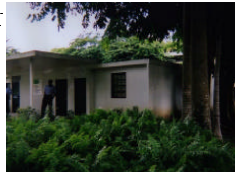
The new office of the RDC Salinas consists of a modern building surrounded by verdant foliage.
